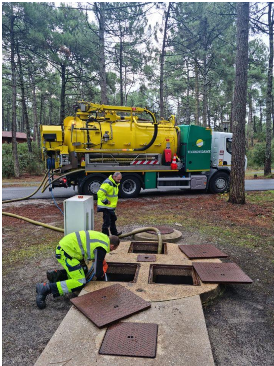
Suction of grease residues in 5 lift wells
