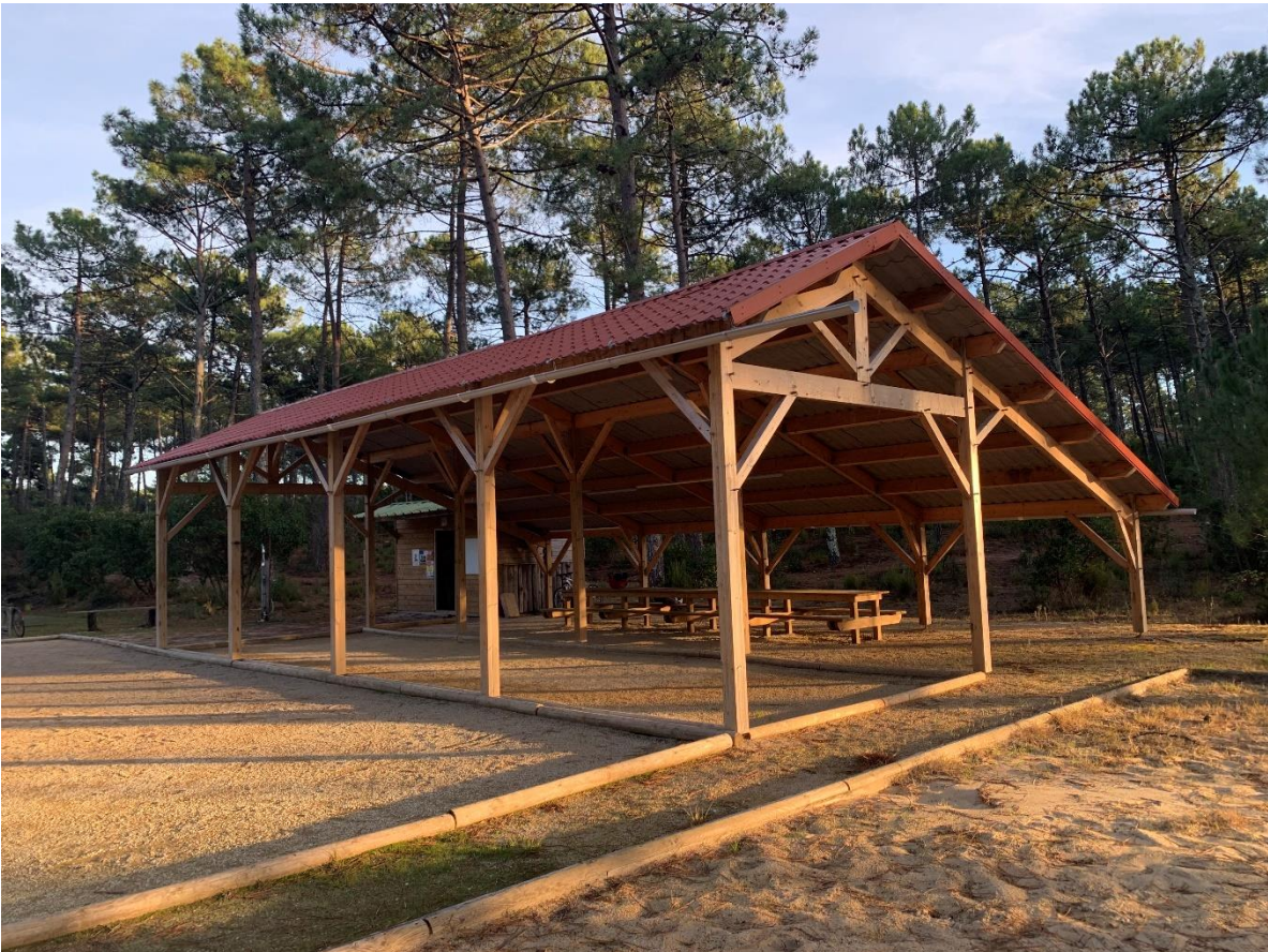
Petanque shelter with gutters, electricity, water, logs and a dining area to gather together
