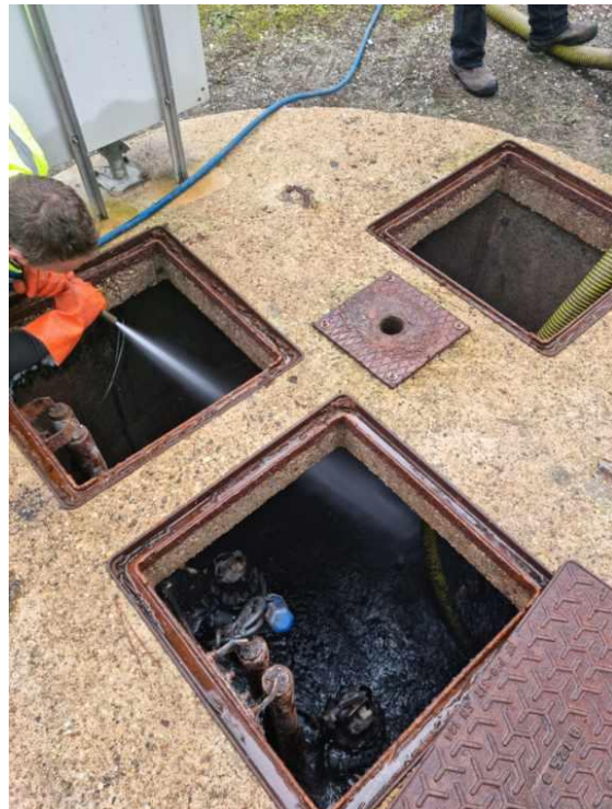
Suction of grease residues in 5 lift wells
